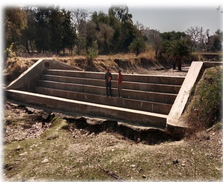
Figure 3 Scouring in Suryavala anicut, Pipalwas Village
